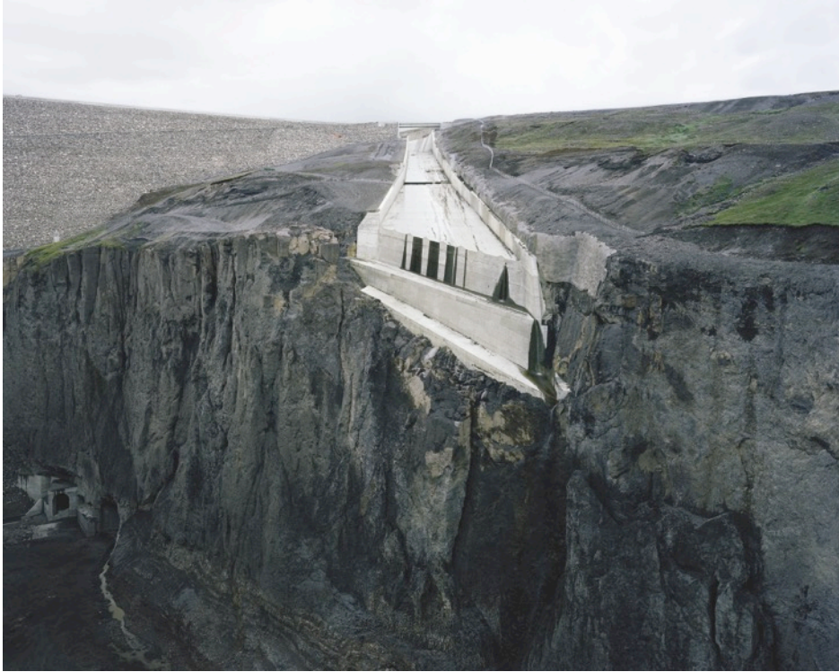
Concrete spillway chute, Kárahnjúkar dam, 2010
